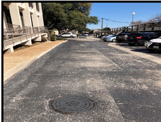
1) SAWS MH# 300155 (to be abandoned) within New 16' Sanitary Sewer Easement (Facing East)
