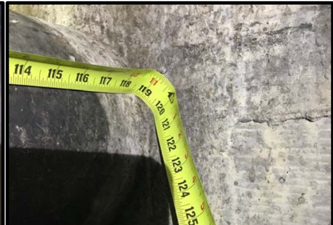
4) Length of Existing Sewer Main Within Storm Box
